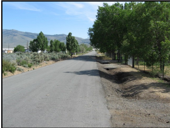
Open ditches, gravel driveways, and little or no street lighting characterize this street in “old” Cold Springs.
