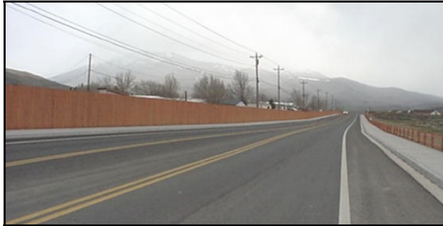
The fencing and lot design shown at left along this arterial should be avoided. The open fencing and/or open space set back shown at right is preferred.
