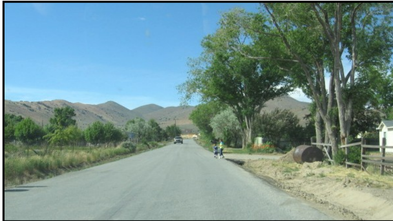
Pedestrians are often forced to walk in the street where open ditches line both sides of the street. Potential conflicts with vehicle use are a concern in such situations.
