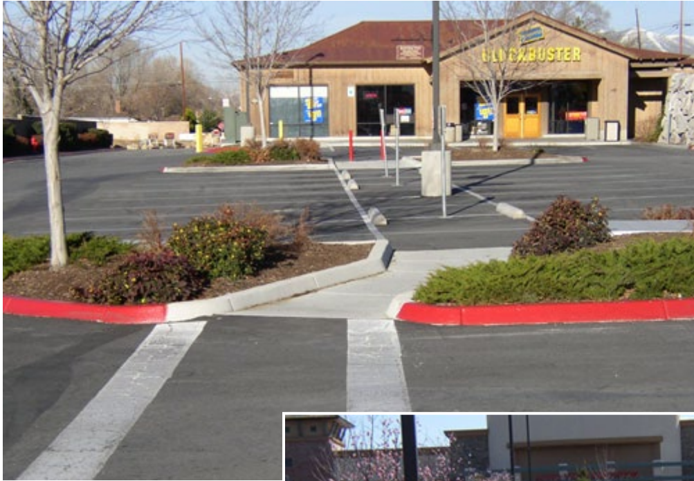
Photo A-1: Pedestrian Walkways within Parking Lots
