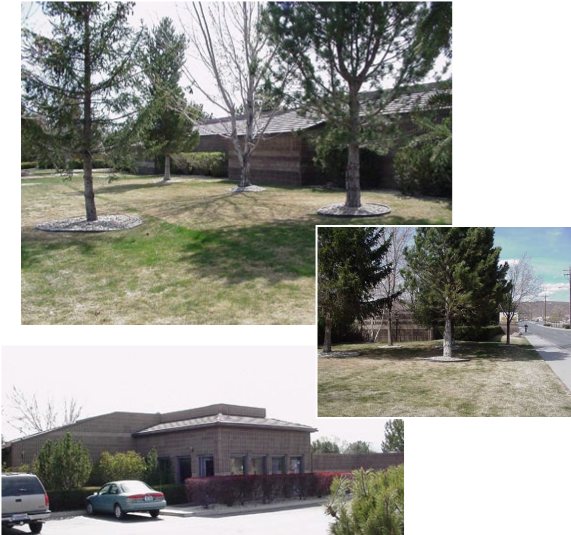
Photo A-3: Desirable Design Characteristics for Personal Storage Facilities
