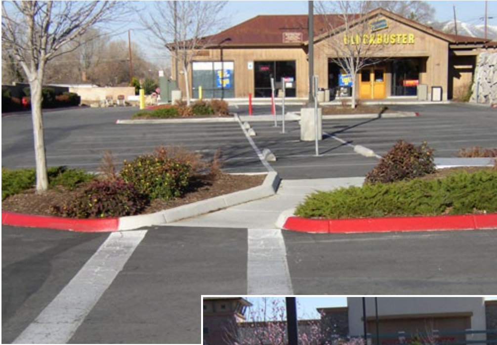
Photo A-2: Pedestrian Walkways within Parking Lots
