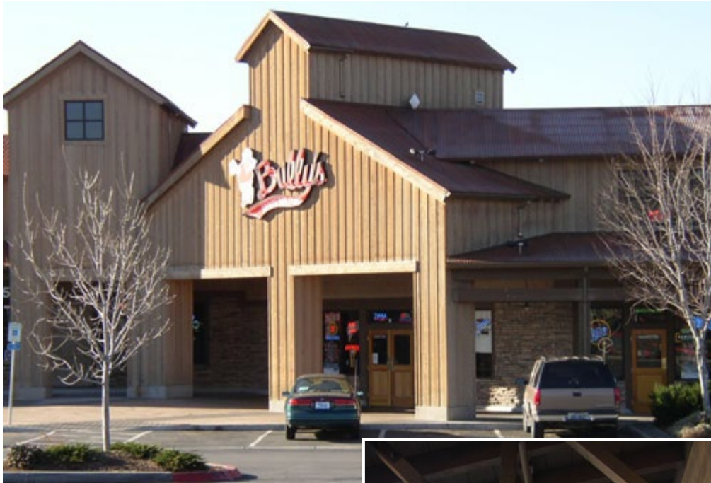
Photo A-2: Representative Architectural Photos
