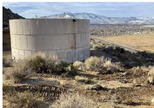
Photograph 2: Top of the Northern Cut Slope
