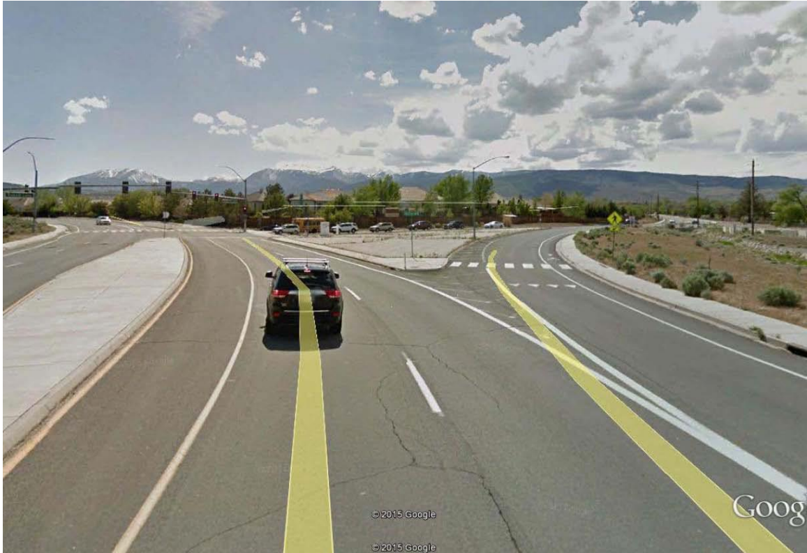
PHOTO OF SITE HEADING WESTBOUND ON ARROWCREEK
