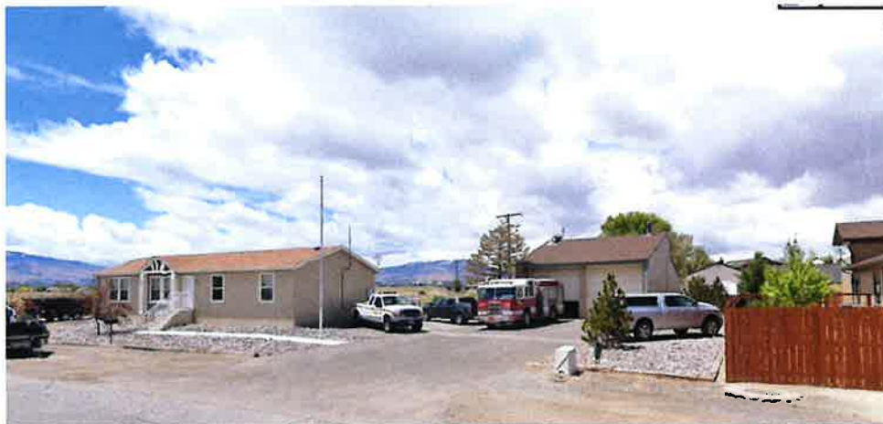
Existing Fire Station #37
