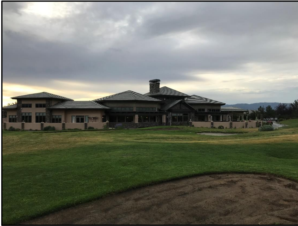
View of the western side of the existing clubhouse building – this portion of building is to remain with additions on the north and south sides.
