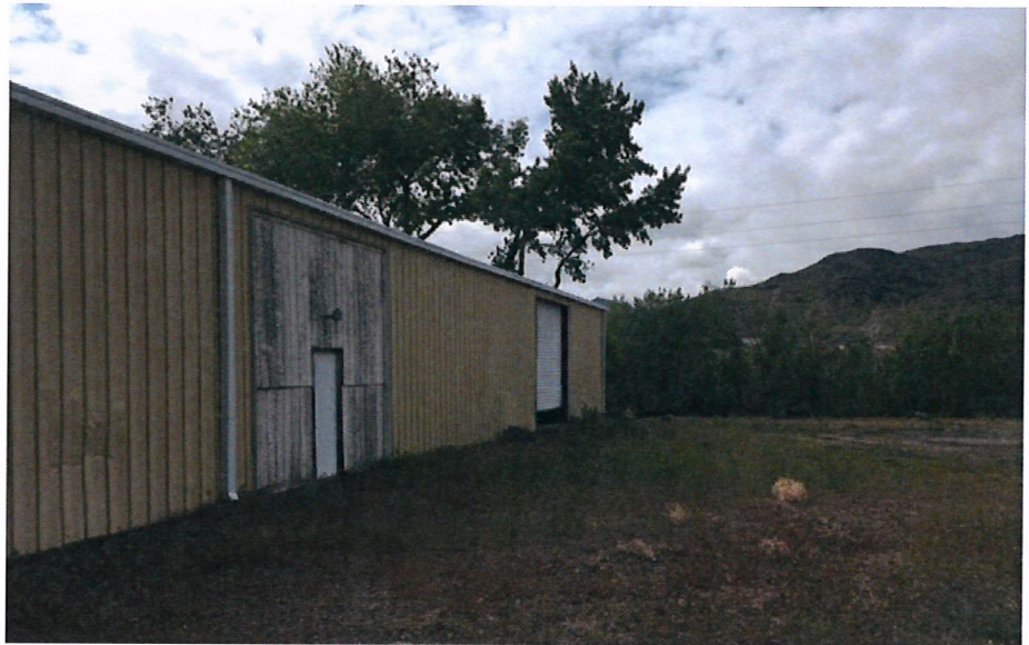
Existing industrial building
