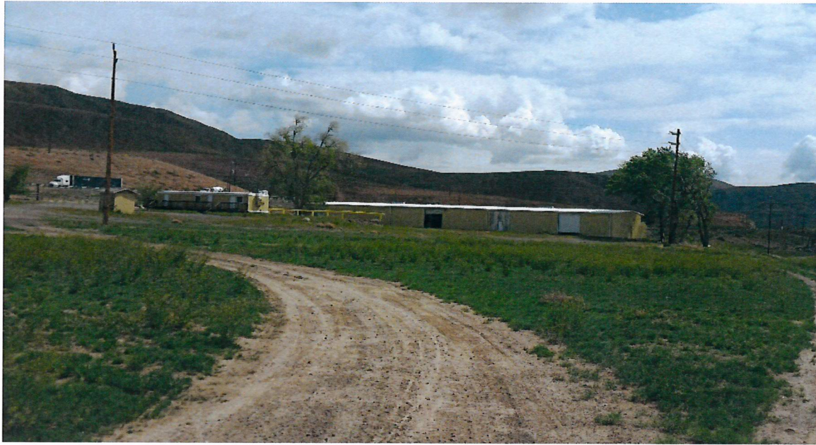
Looking northeast across site with freeway in background
