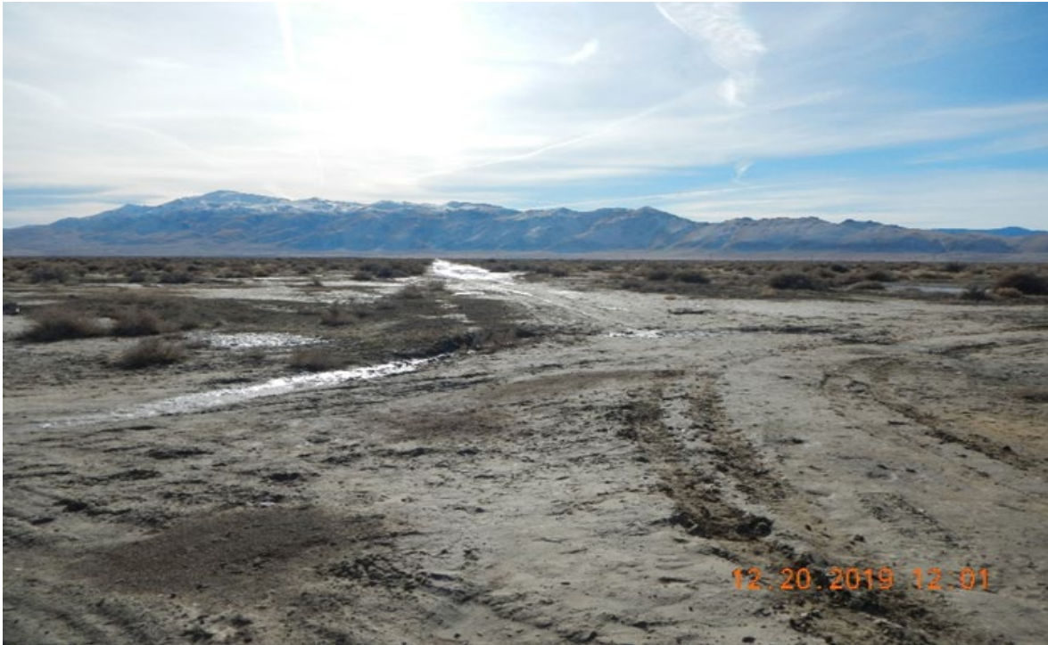
Photo 4: View south down Calneva Road just after rain with water collecting in low spots of road.
