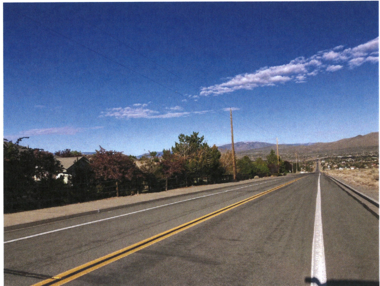
View toward the west of La Posada Drive improvements.
