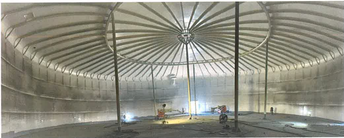
Photo: Pyramid Tank Rehab Project
